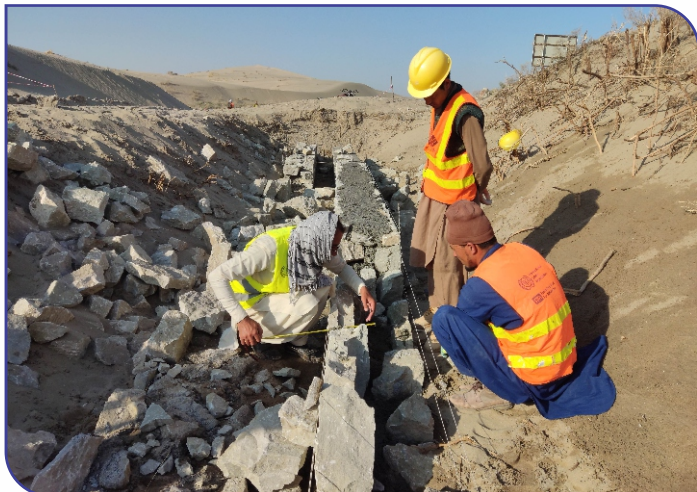
Figure 1: Stone Masonry Side Drain Construction in Shortepa District Road.
