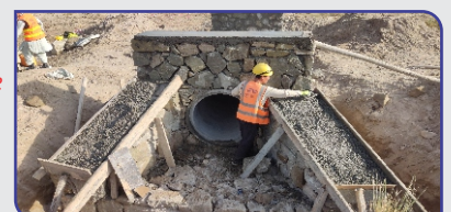
Figure 2: Cross Drainage Structure Construction in Rehabilitation of Shortepa District Road
