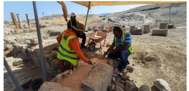
Rehabilitation works at Pella Site
