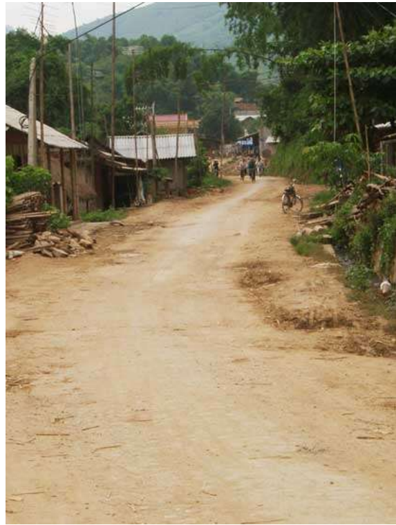
End of selected road section on NH 15
