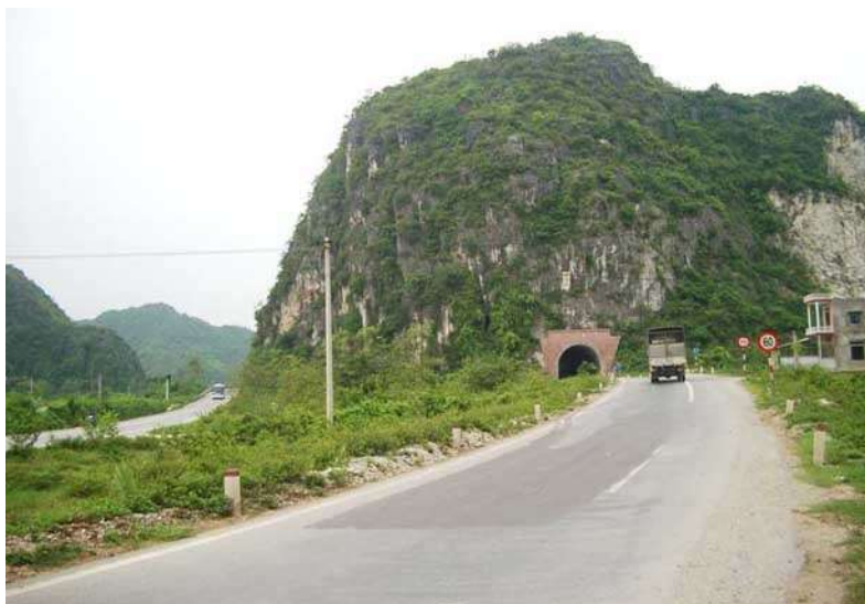
Section of NH 1 south out Hanoi with dual carriage way, also selected as part of the first year maintenance programme.
