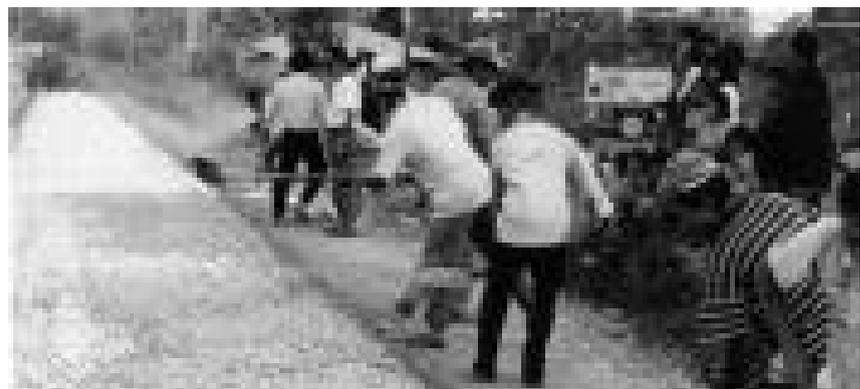
Bitumen seal work using labour-based techniques
