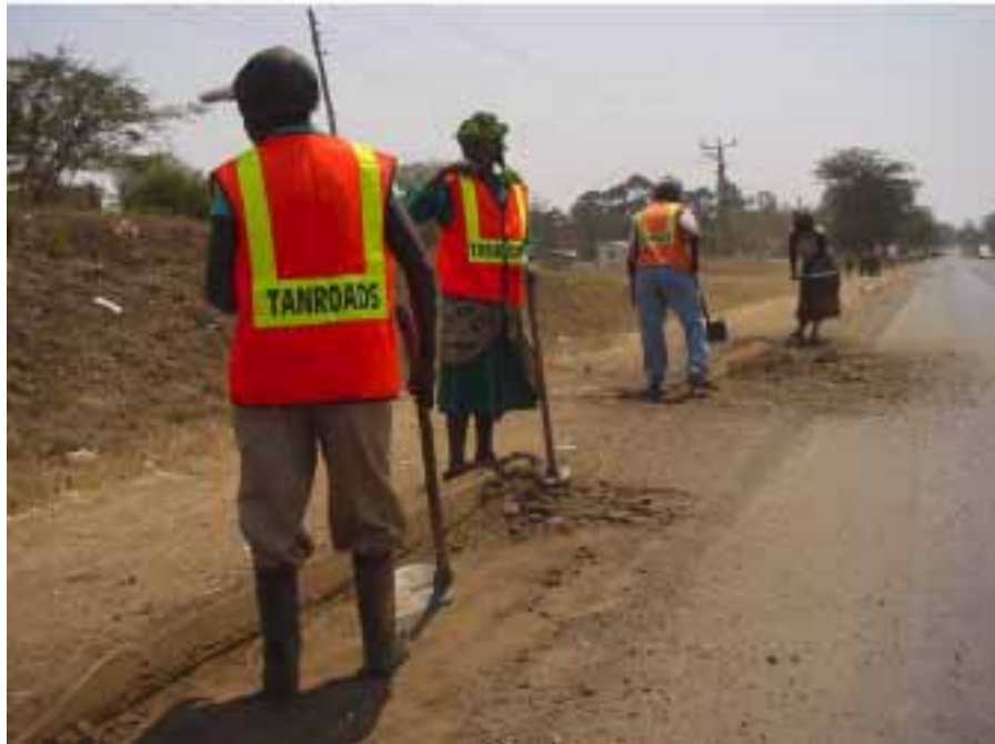
Site visit - TANROADS
