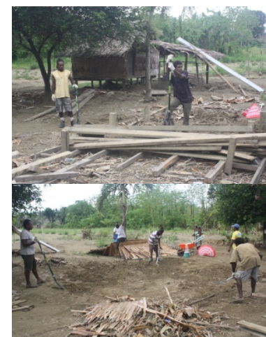
FIGURE 4. THE WORK BEGIN!
