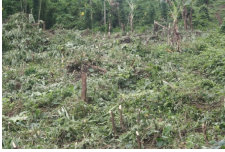
Newly cleared sight for community relocation in Papangu.
