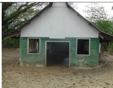
Flooded and damaged community hall in Roroni
