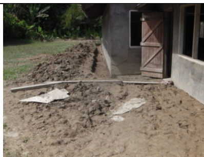
Drains being dug around a church in Roroni Community.
