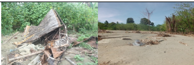
Destroyed houses and shelter than needs to be rebuilt. On the left the remains of a group of houses in Papangu.
