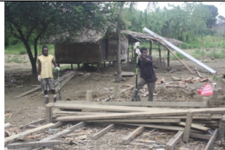
Rebuilding community infrastructure and houses in Papangu.
