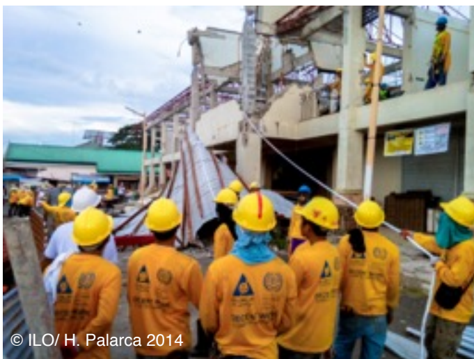
Workers are safeguarded by personal protective equipment (PPE) as they pull down the damaged roof of Loon's public market.
