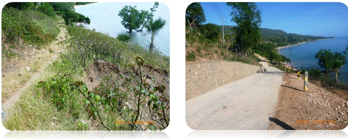
Photo 4: Condition of the Boile-Uatabo Road, before and after the Road Rehabilitation
