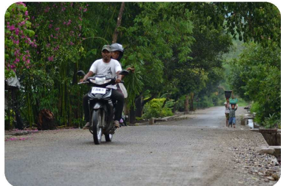
Penetration Macadam Surfacing, Maliana-Saburai
