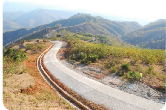
Plum Concrete Surfacing, Mahata-Kusi
