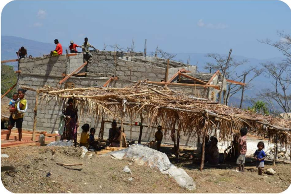
New house in Aldeia Cassal, Maliana-Saburai road
