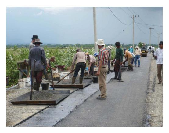
For above reasons the project introduced a bitumen emulsion technology (sometimes also referred to as 'cold asphalt'). This environmentally-friendly and durable technology has been successfully applied in other countries and the initial findings on the demonstration sites in Aceh reveal that this approach produces a quality road.
