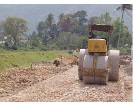
PWD and the project also used Latasir (a sand/bitumen mix) as a wearing course number on а roads. The available information indicates that the costs per kilometer were lower for roads constructed by the project with this wearing course, compared to costs of construction undertaken by PWD.<sup>5</sup>
