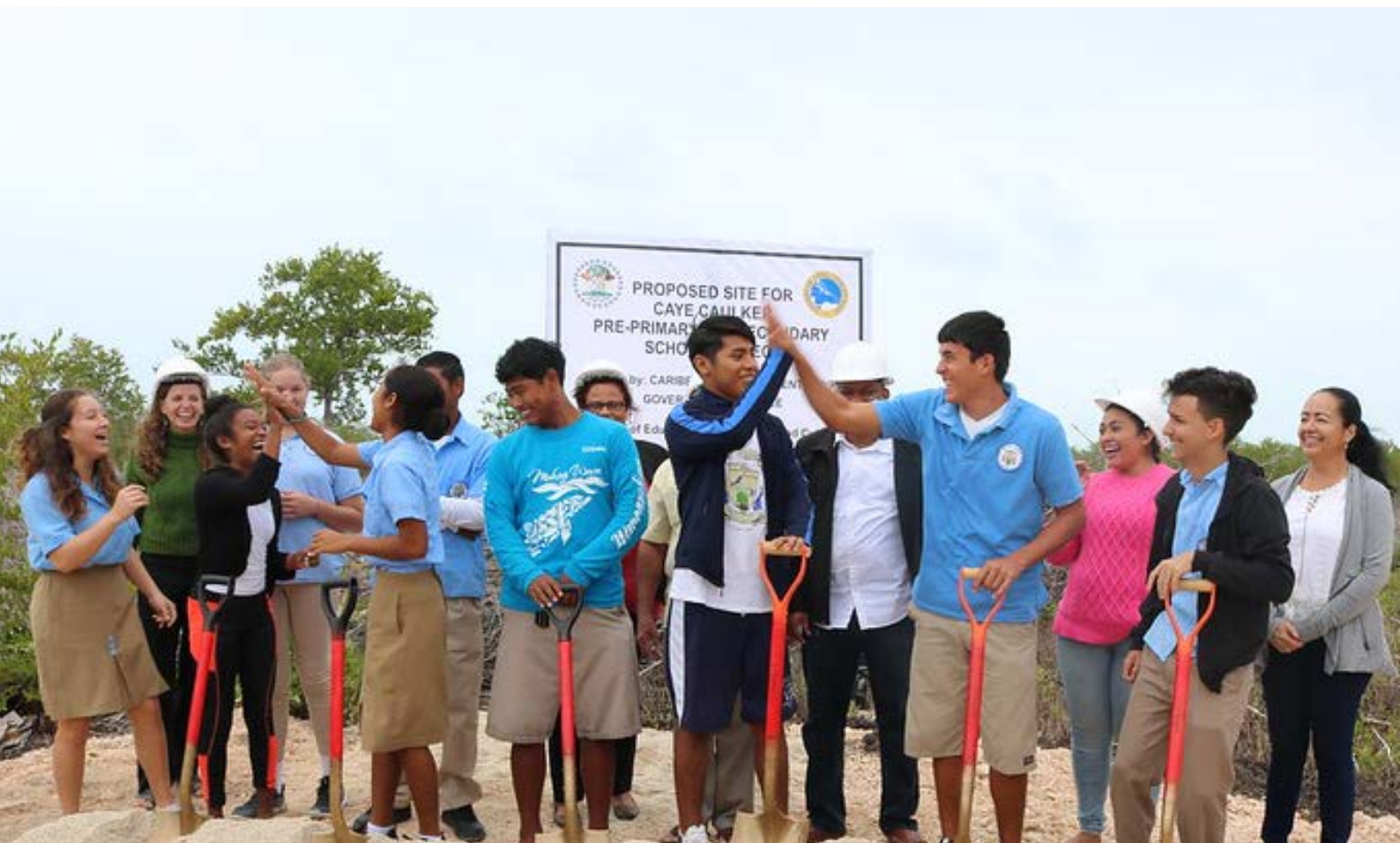
Photo, Government of Belize Press Office: Breaking ground for schools in Caye Caulker and San Pedro, Belize
