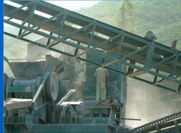
UNGUARDED MACHINES, DUST, WRONG FOOTWEAR, NO PPE
