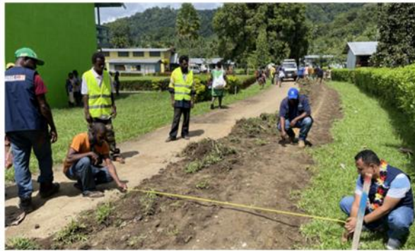
Exhibit 14 Setting out for the Banak – Wautogik road rehabilitation and maintenance in East Sepik
