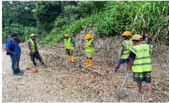
Exhibit 11 RMG workers engaged in road maintenance
