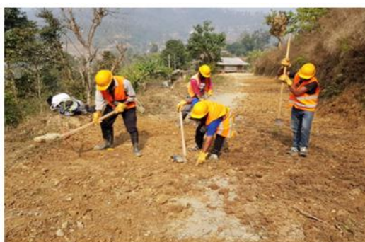
Exhibit 9 Routine road maintenance by RMG workers
