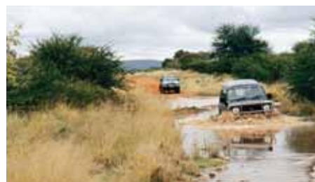
Roads without maintenance
