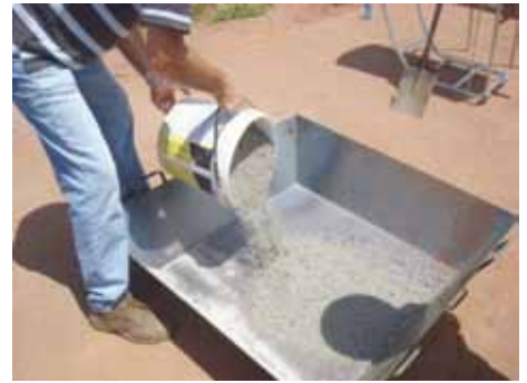
Batching of aggregates
