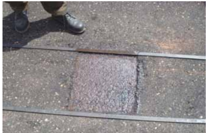
Area prepared for placing of asphalt
