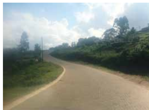
Completed block-paved sections
