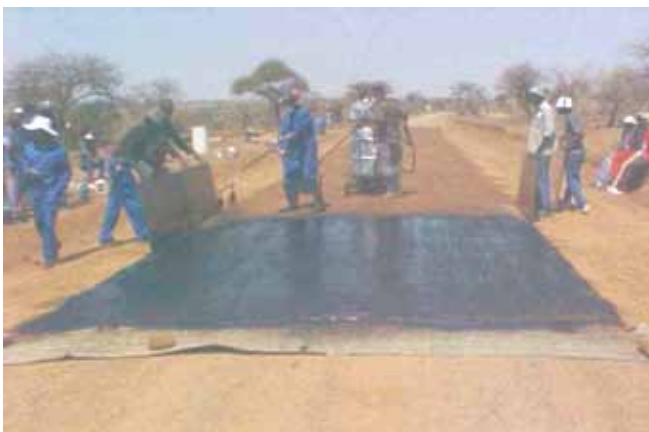
Spraying using protective screens and reinforced paper
