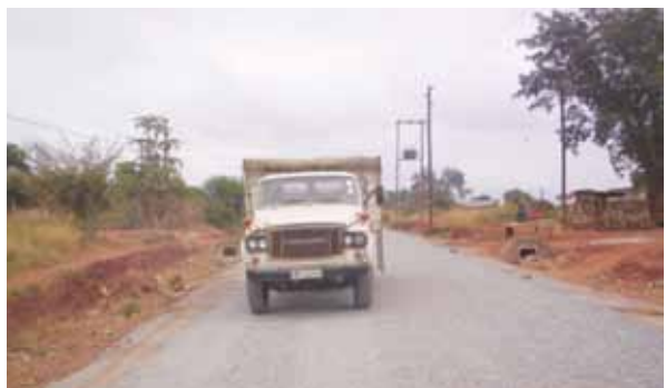
Loaded Tipper Trucks assisting in compaction
