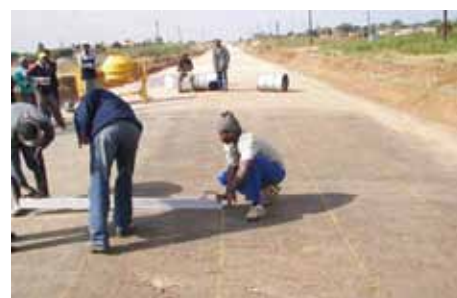
Marking position of guard rails
