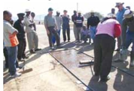
Application of tack coat
