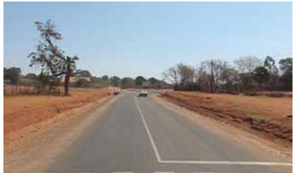
A completed Otta Seal section
