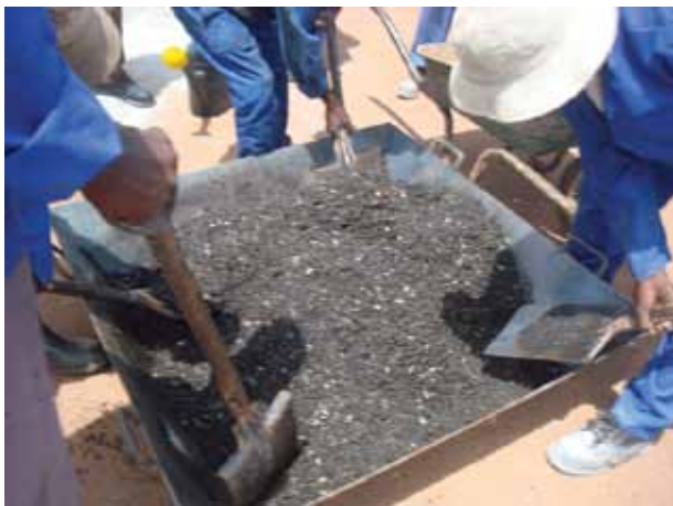
In-situ hand-mixing of asphalt
