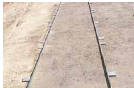
Placing the guard rails
