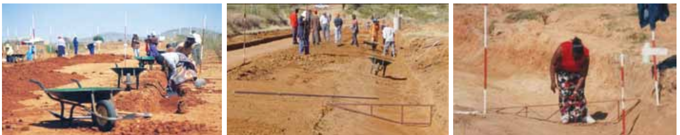
Constructing open drains using labour-based work methods
