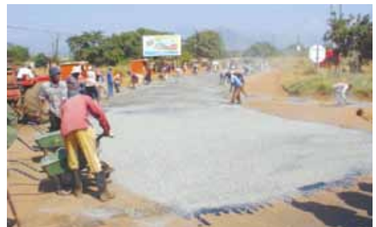
Slow spreading rate of aggregates by hand
