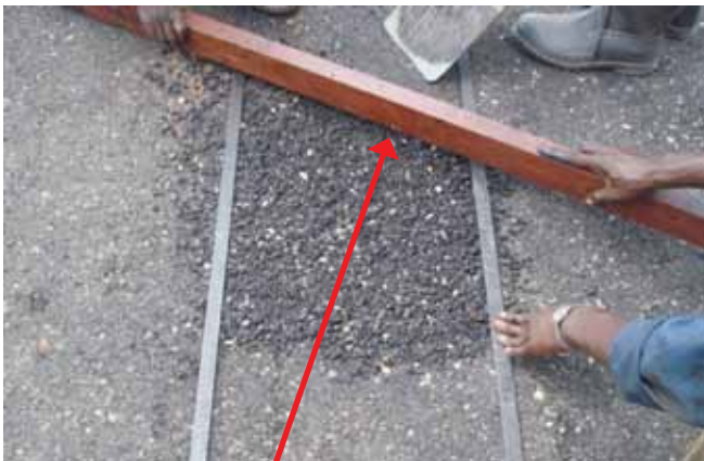
Screed the top
