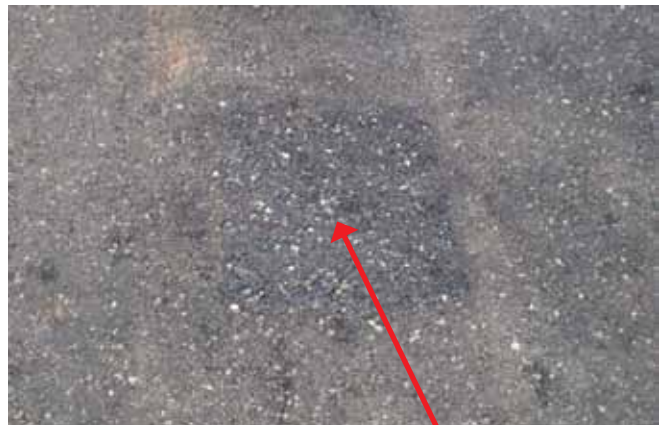
Finished "patch" hardly visible
