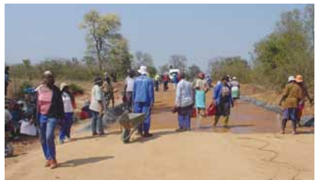
Watering the base Surface
