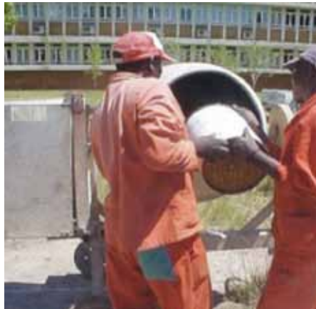
Feeding aggregate, lime and cement into mixer
