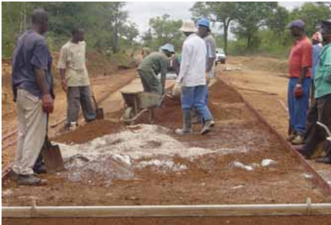
Lime stabilization in practice
