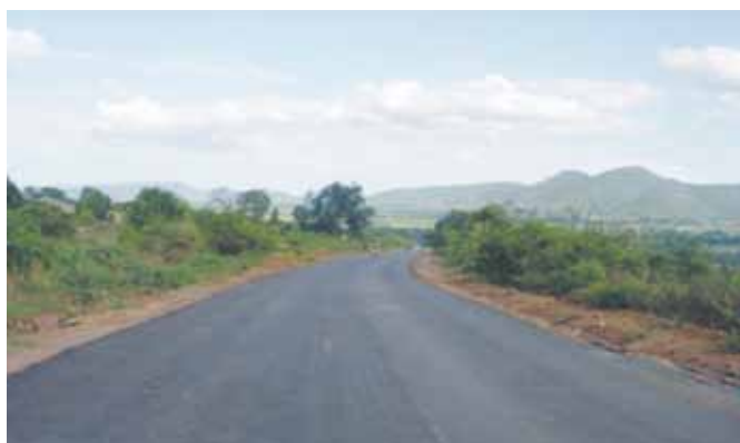
Completed asphalt sealed sections
