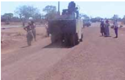
Compacting Otta Seal natural gravel
