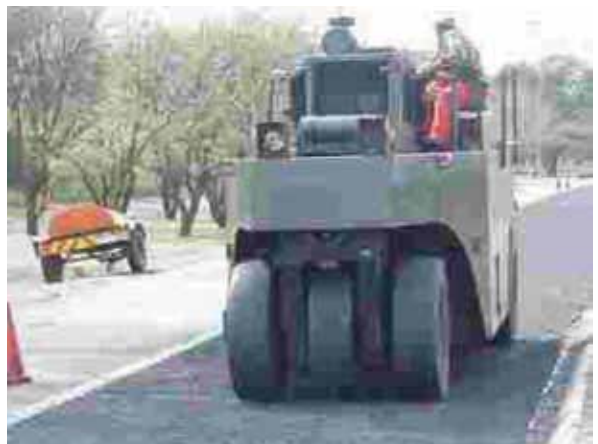
Compaction by a Pneumatic Roller
