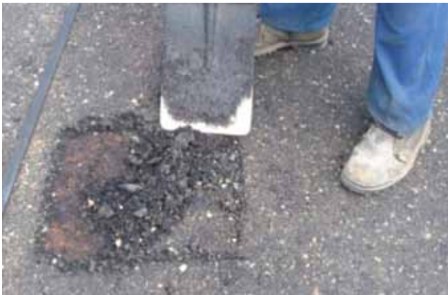
Removal of old material
