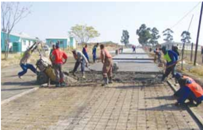
Laying of ultra-thin concrete
