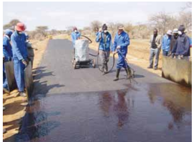
Spraying operation in practice
