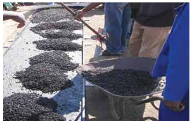
Spotting the asphalt
