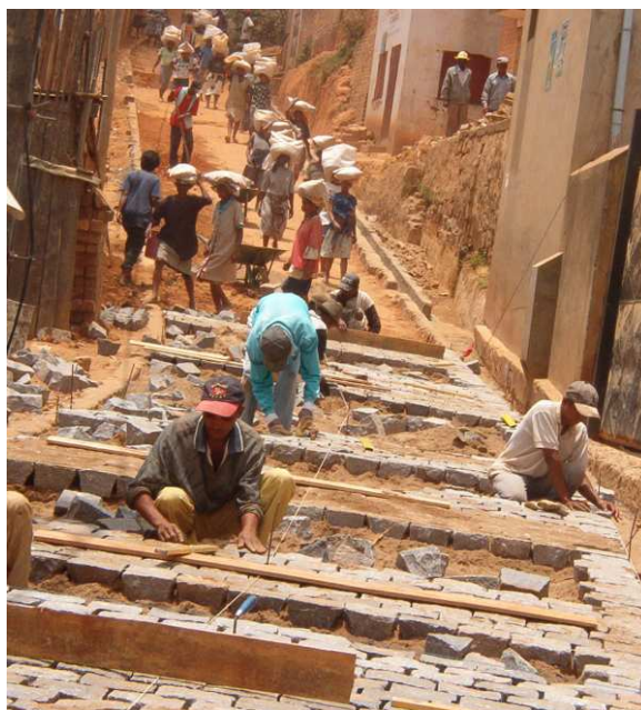
Madagascar: Paving of a 533 meter long road in Ambohitafy (Antananarivo province). Photo: Marc van Imschoot
