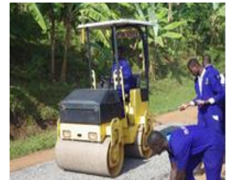
Partially using equipment like 1t vibration roller
