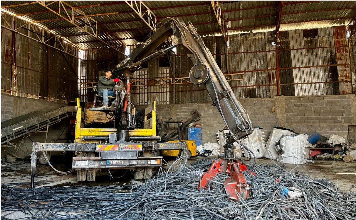
Photo 5.5 Farmland irrigation pipes transported for washing and crushing
