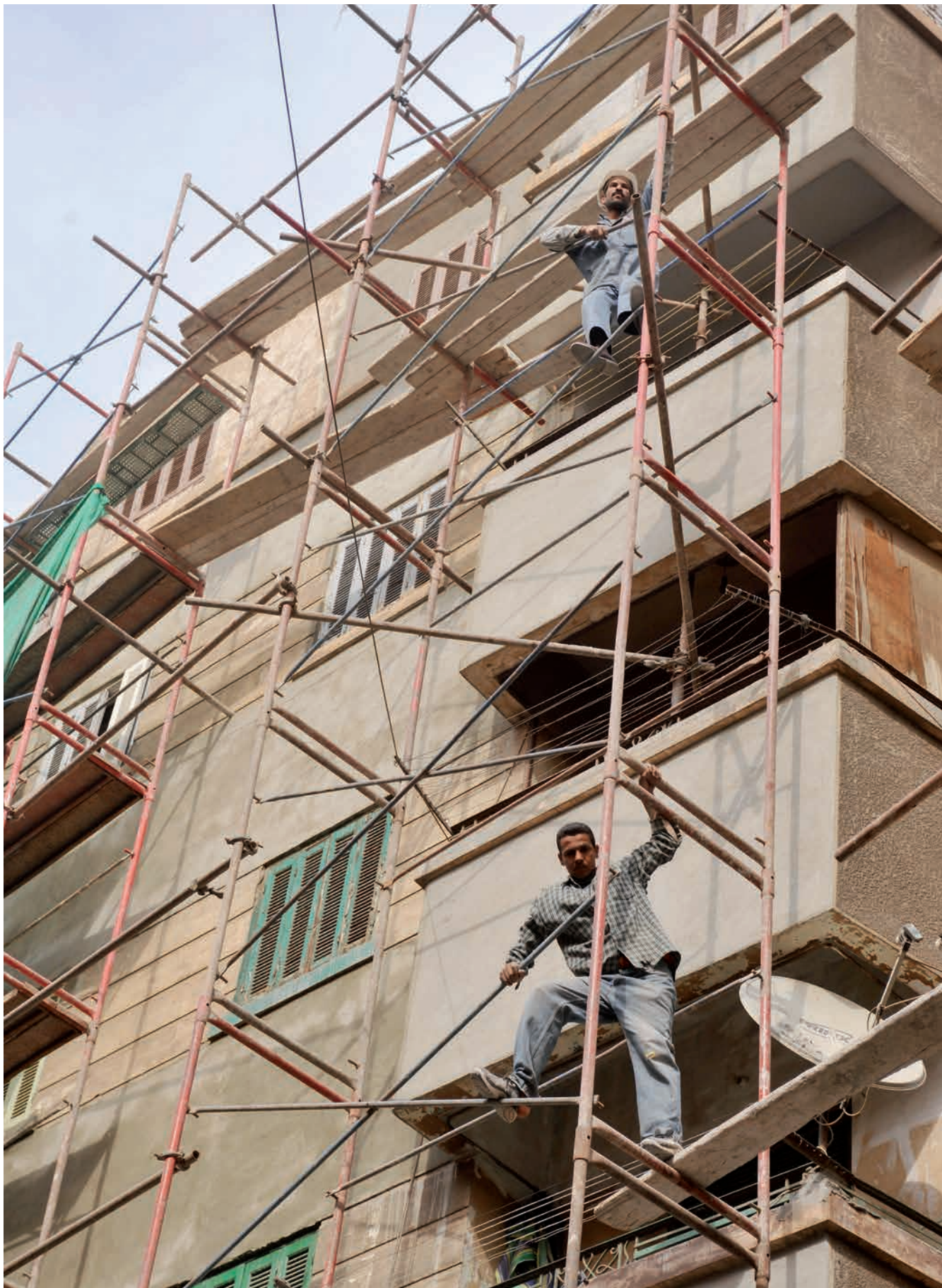
Construction workers, Cairo, Egypt.
