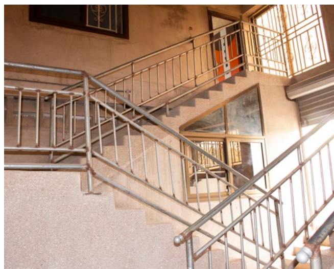
After: railings installed company wide for user safety
