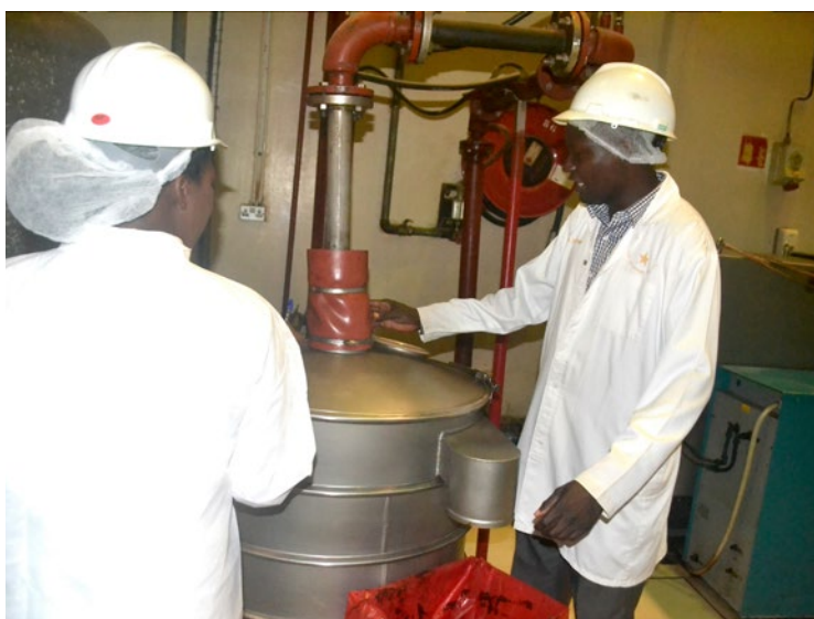
Rafat Kasin, Project Coordinator, describing a project to reduce leaks
