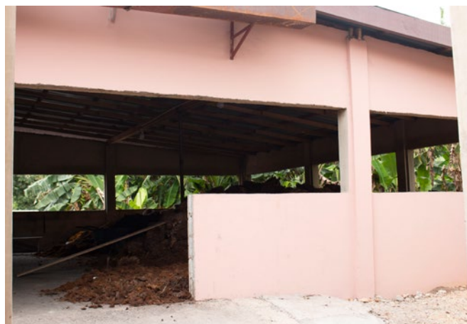
After: Fibre residue now stored in a proper structure
