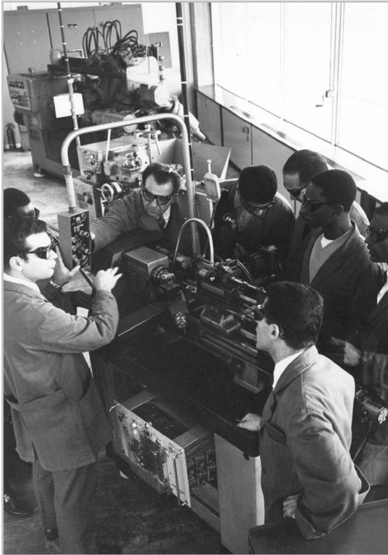
A Turin Centre Training Course, February 1969. A multi-lingual instructor explains the operation of a modern automatic lathe, run on an electro-pneumatic system, of the type used in making components for the automobile industry.
