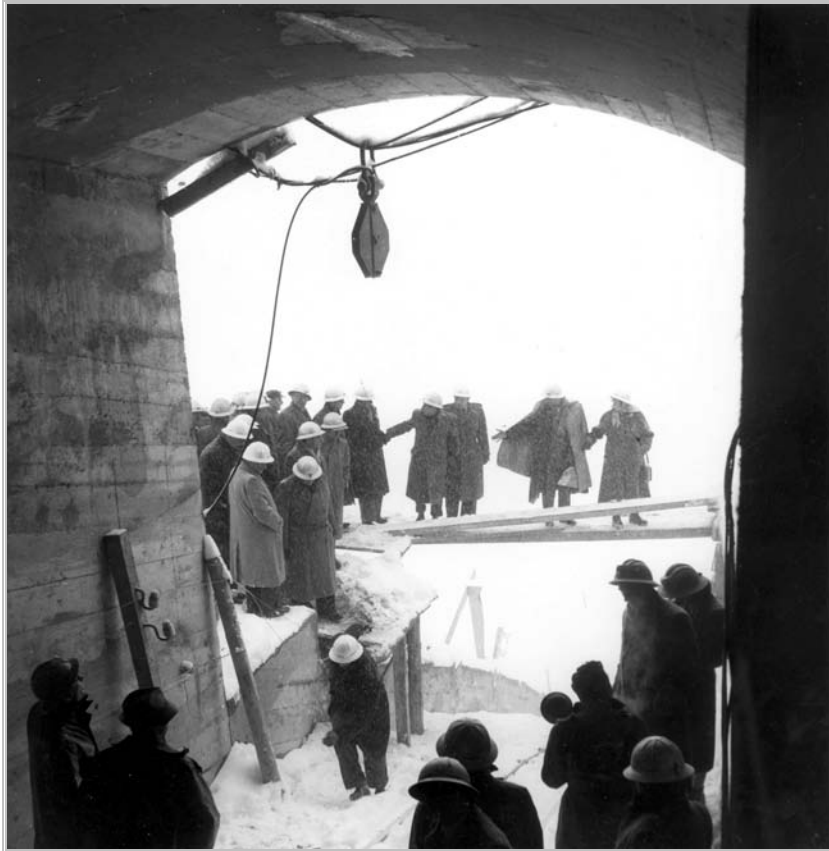
Delegates to the 4th meeting of the Building, Civil Engineering and Public Works Committee (26 October – 6 November 1953) visit the construction site of the Grand Dixence Hydroelectric Dam in Valais (Switzerland).
