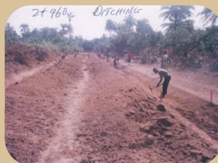
Ditching and preparing the road
