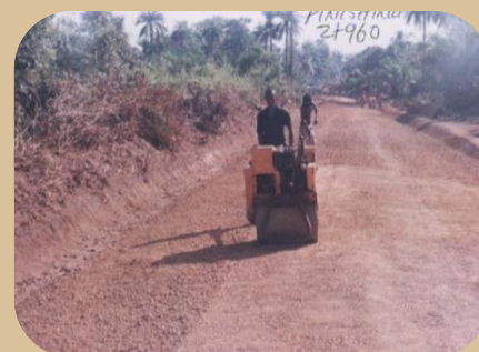
Compaction after spreading and watering
