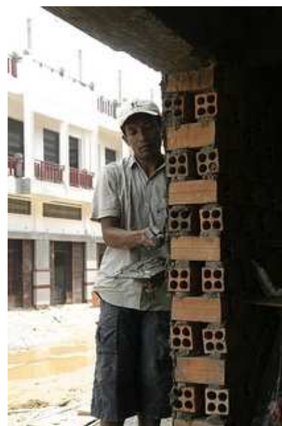
Construction Worker, Cambodia © ILO
