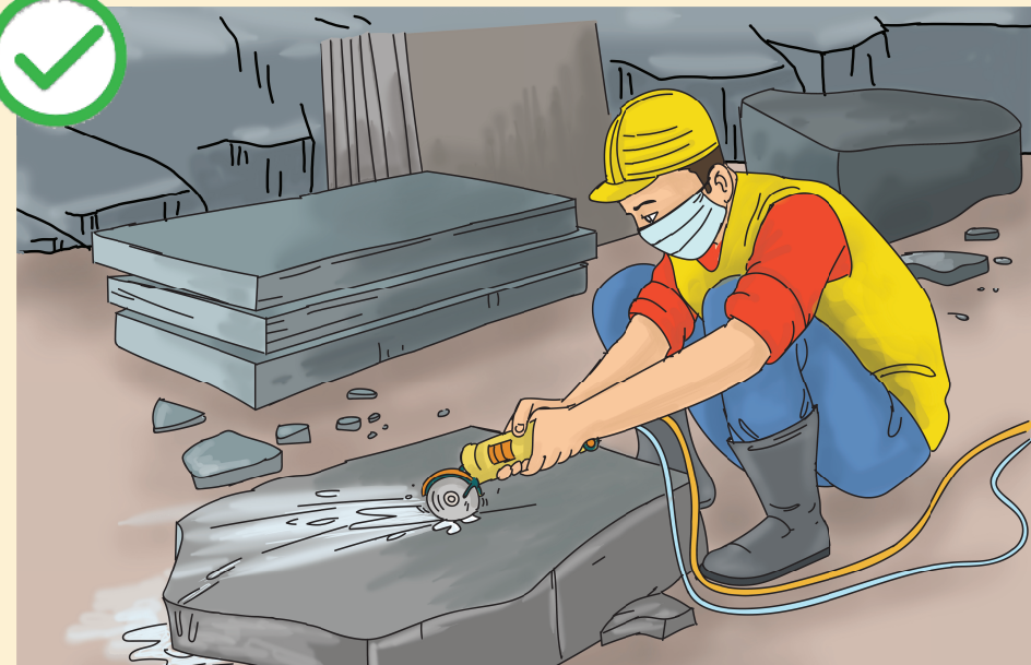
Reduced dust emission with water jet
