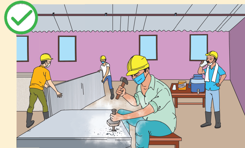
Provide protection from the sun and provide portable drinking water
