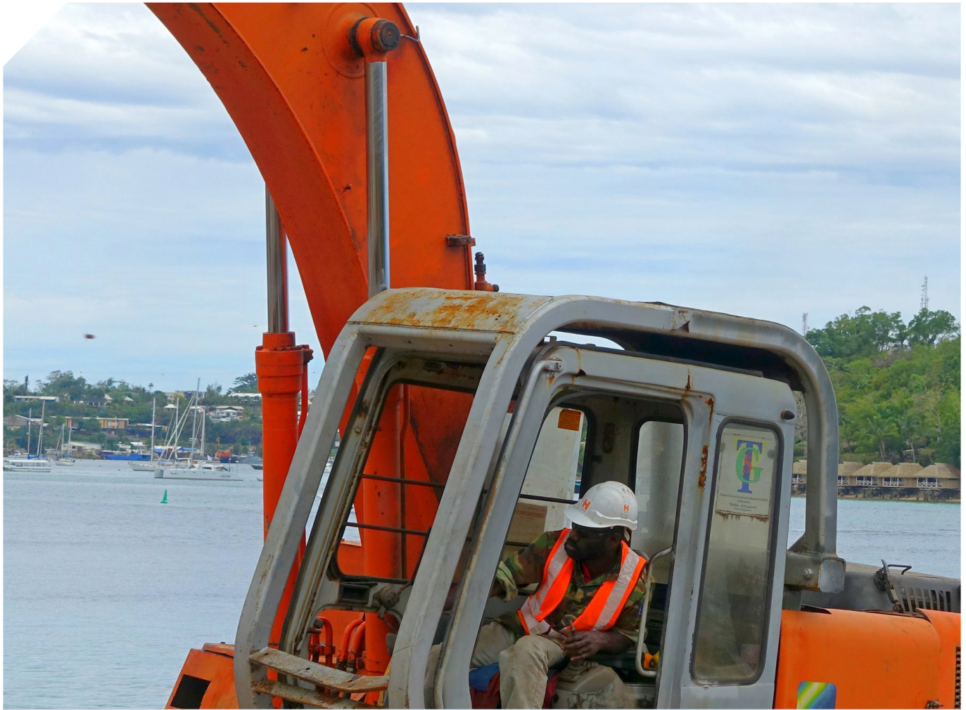
Seawall maintenance in Port Vila, Vanuatu. ©CO-Suva/ILO
