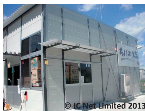
© IC Net Limited 2013 Temporary factory of Chiba Seaweed Store
