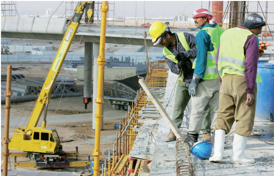
Construction workers, Gulf Region
