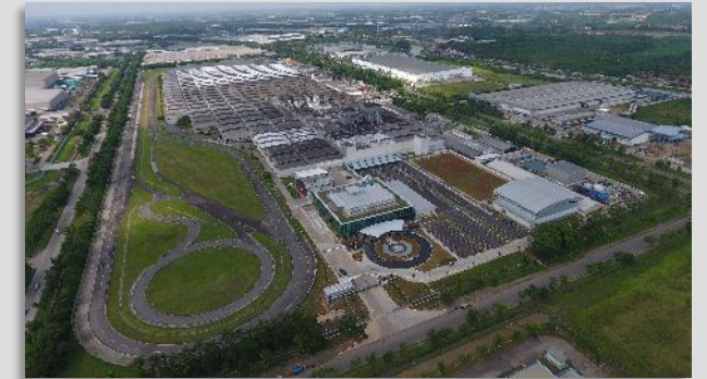
BSIN Head Office and Karawang Plant
