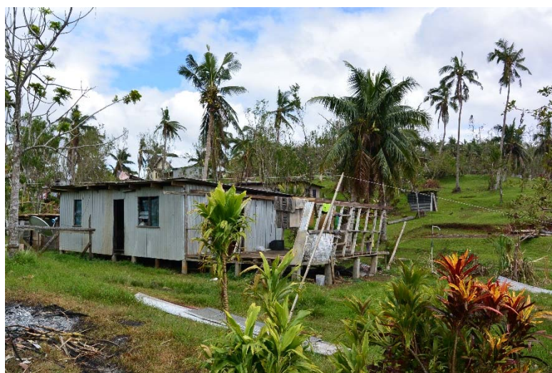
Houses damaged in one of the target communities.
