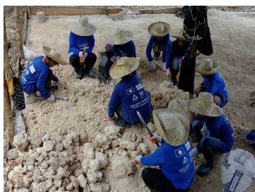
Limestone, which is abundant in the area, serves as the main raw material in making ICEB.
