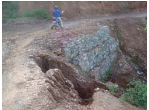
Cut in road shoulder
