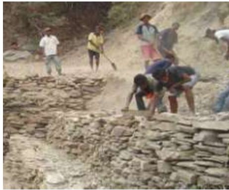
Stone masonry for slope protection
