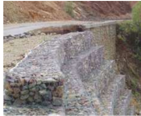
Slope erosion repair by using gabions
