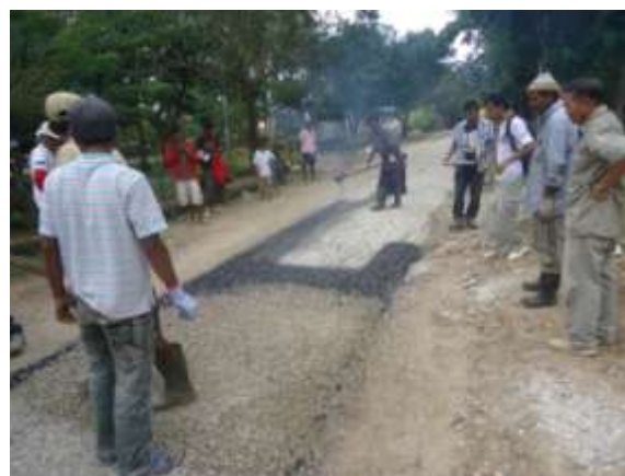
Aggregate layers – base, intermediate and surface
