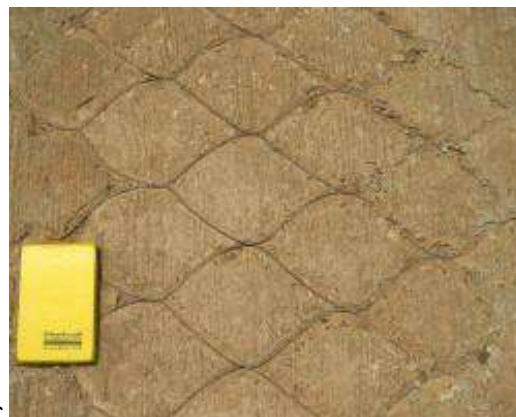
Geo-cells 2 years after construction
