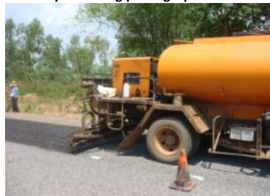
Spray run marked with guide for driver
