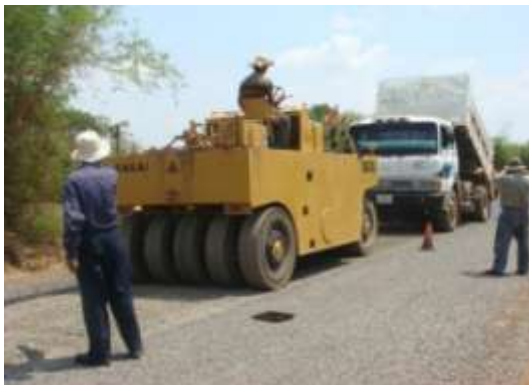
Rolling follows immediately after placement of stone chippings
