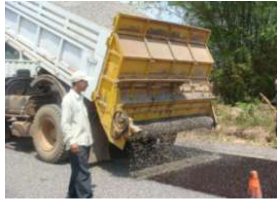
Mechanical spreader and speed of truck governs application
