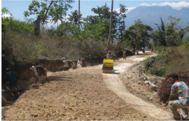
Picture 8: Compacting while maintaining camber
