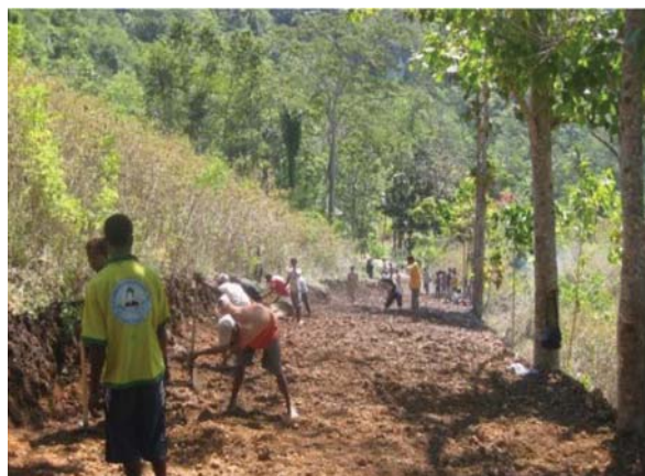
Picture 5: Cutting and leveling
