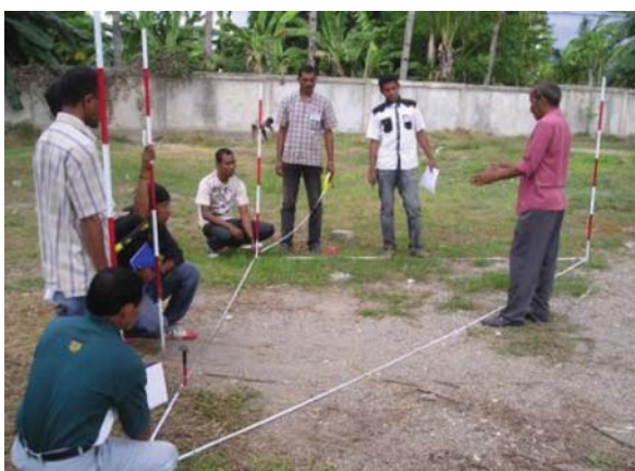
Picture 3: Setting out 90° angle from centre line
