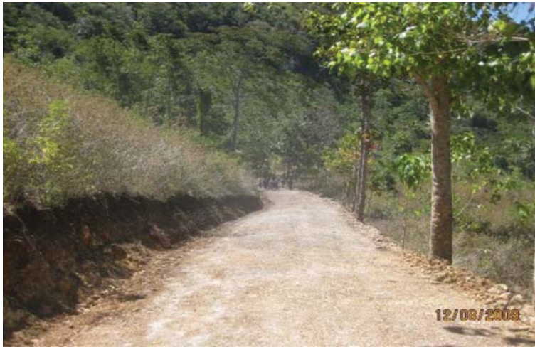
Picture 7: Completed camber of gravel road
