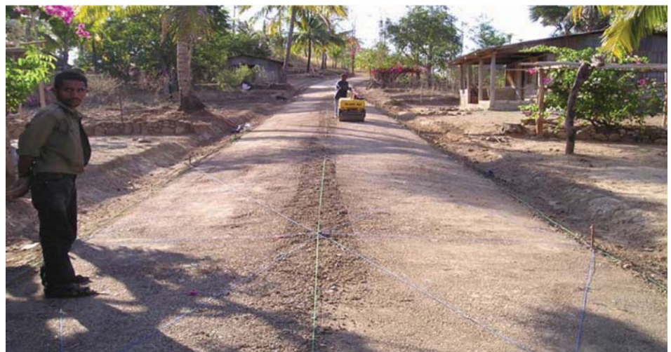
Picture 9: Checking the camber using pegs and strings
