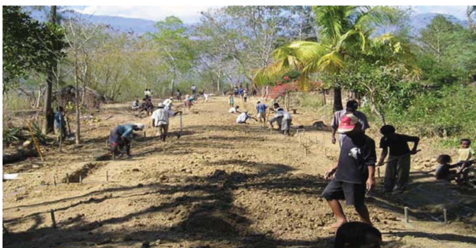
Picture 6 : Constructing camber with soils from side drains
