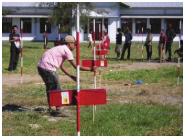
Picture 2: Setting out straight lines and gradients
