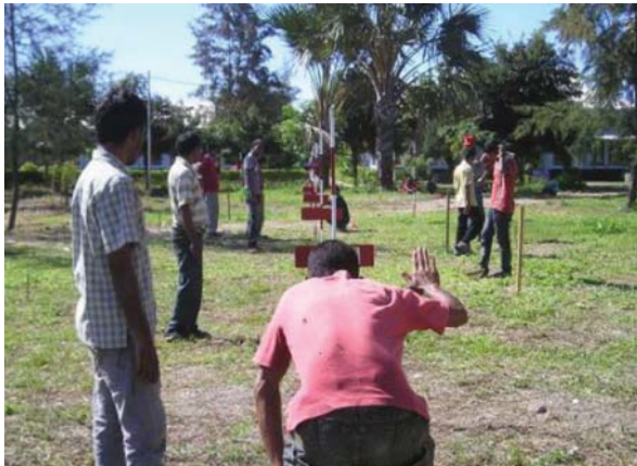
Picture 4: Checking gradient along center line
