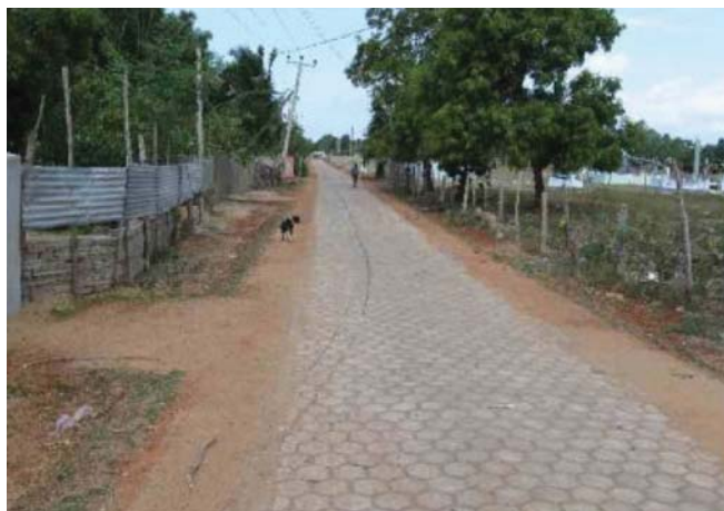
Gambar 24: Concrete block pavement
