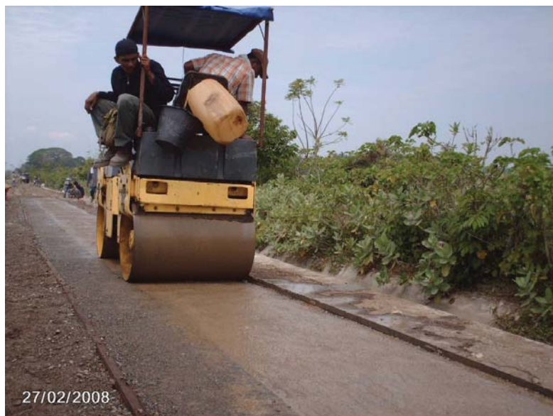
Gambar 37: Compaction of base-course for cold mix sealing
