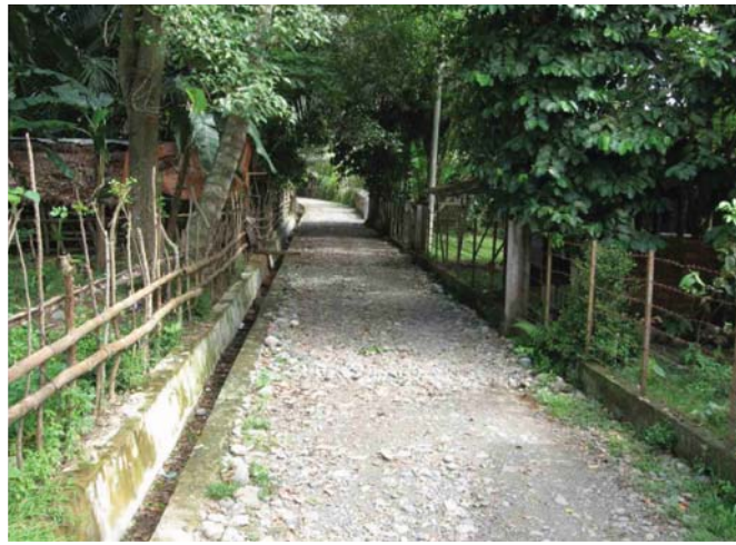
Gambar 27: Telford after some years of operation
