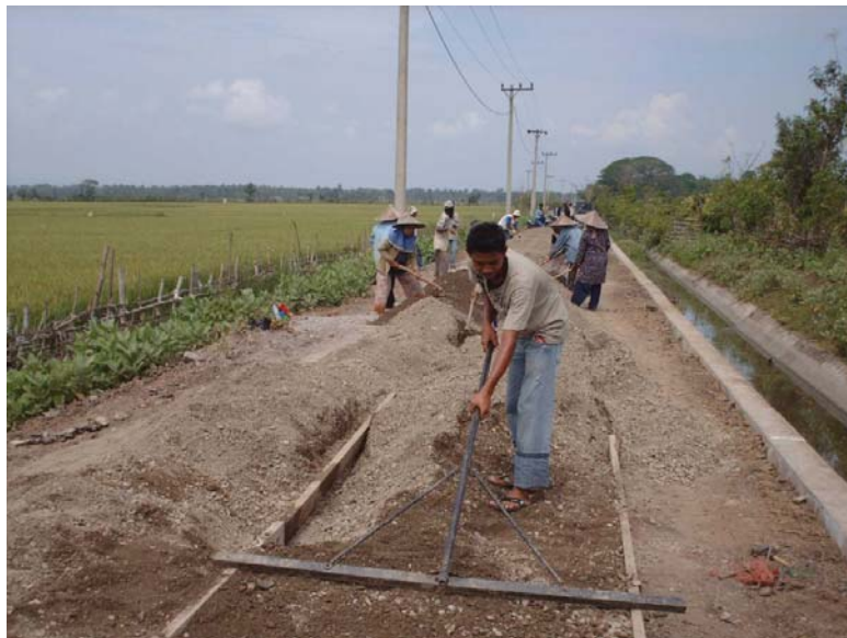
Gambar 36: Spreading aggregates for base-course using steel shutters for form work
