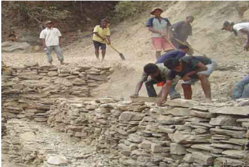
Gambar 33: Dry stone retaining wall under construction
