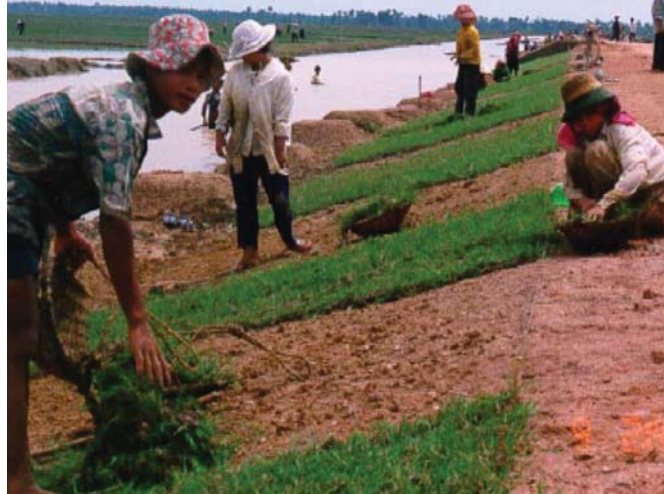
Gambar 31: Turfing of side slopes
