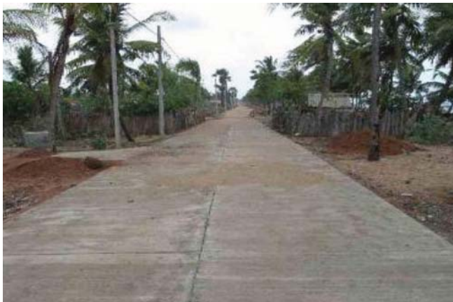
Gambar 26: Completed concrete road
