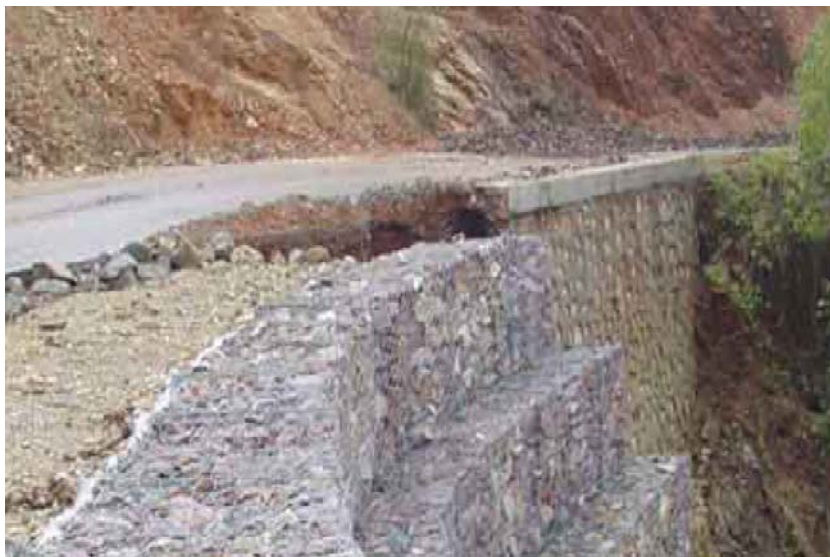
Picture 34: Gabion retaining wall
