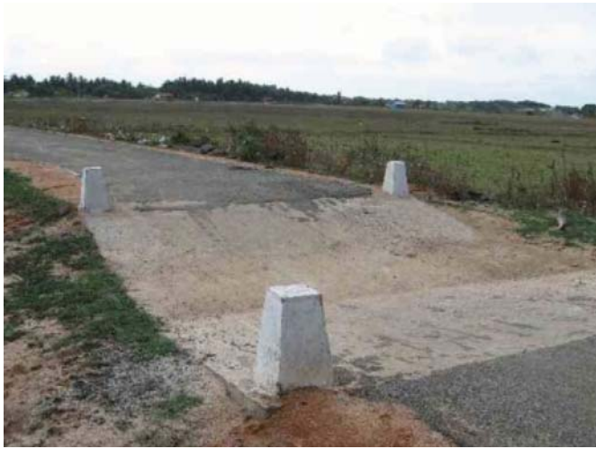
Gambar 16: Example of concrete drift
