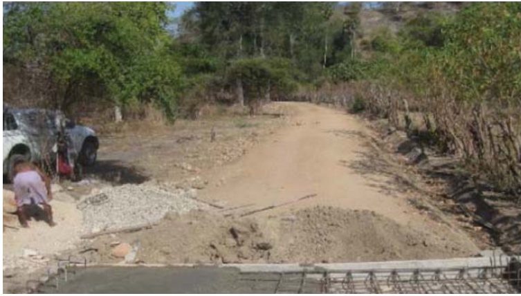
Gambar 19: Construction of box culvert
