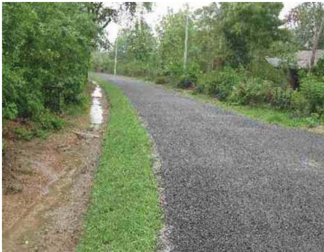
Gambar 30: Grass protection of shoulders
