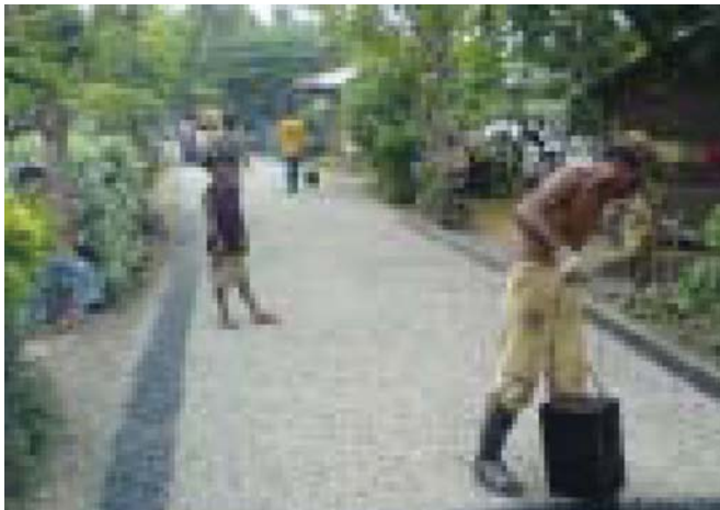
Gambar 29: Spraying bitumen for Penetration Macadam
