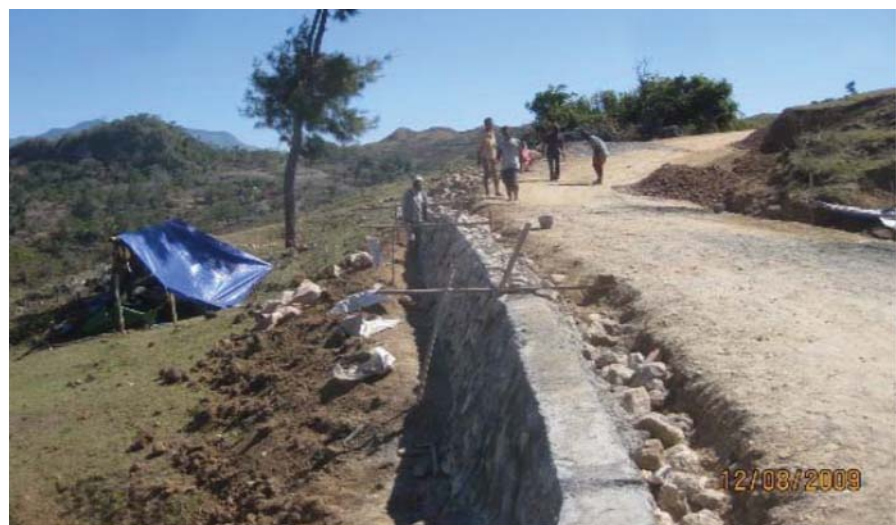
Gambar 32: Masonry retaining wall
