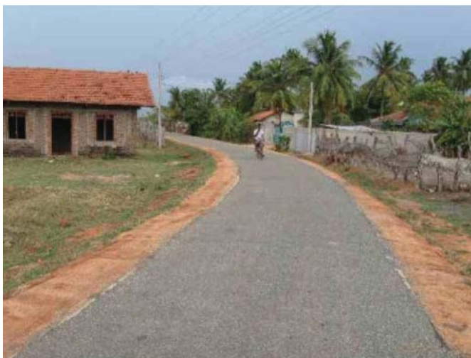
Gambar 28: Road with DBST Surface
