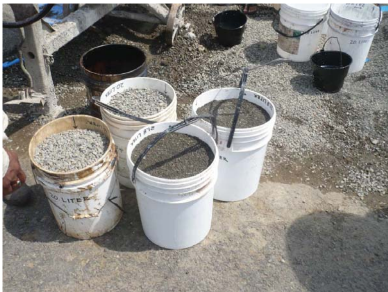
Gambar 38: Measuring aggregates for mixing cold mix
