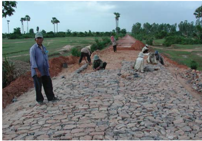
Gambar 25: Stone pavement road
