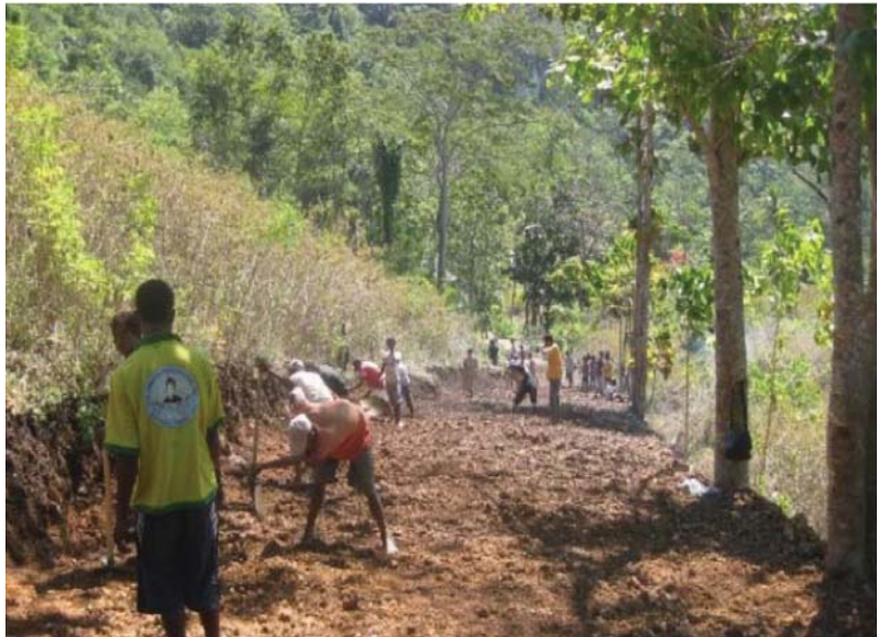
Picture 5: Cutting and leveling
