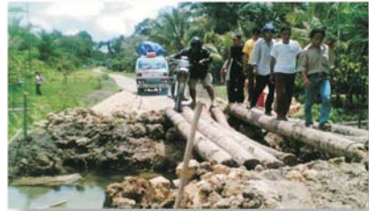
Temporary bridge in Nias that would need to be permanent.
