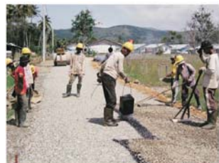
Surfacing in Aceh Besar
