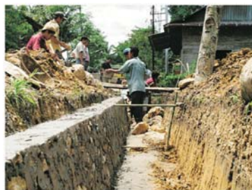
Training and supervision during rehabilitation
