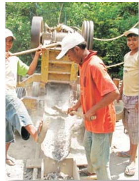
“Producing” materials on site.
