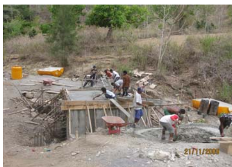
Ossurua, Viqueque during construction
