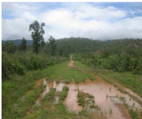
Fahilebo, Liquica Before rehabilitation
