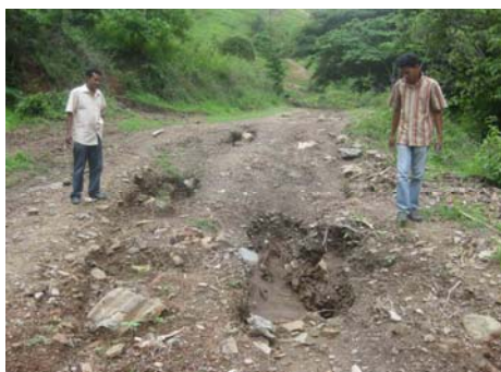
Bedquira, Metinaro before rehabilitation
