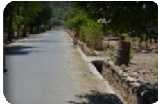
Slabs are constructed across drains to facilitate access for people with disabilities Konstrui ona palas hirak iha baxeta hodi bele aksesu ba ema ho kondisaun defisient
