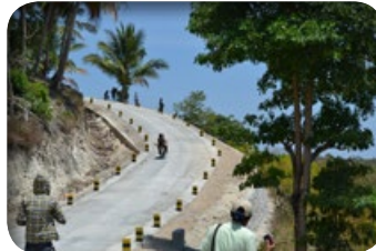
R4D rehabilitated road, Balibo-Cowa (10 Km), Bobonaro District: Another example of concrete pavement on a section with a steep road gradient Distritu Bobonaro, R4D reabilita ona estrada Balibo-Cowa (Km 10): Ezemplu seluk ida husi trotoar betuun iha sekaun ida ho gradienti estrada nai naruk
