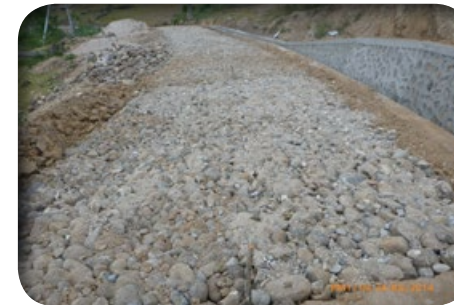
Completed Telford section on R4D road Kompleta ona seksaun Telford iha estrada R4D
