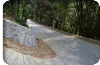
R4D rehabilitated road, Lianai-Grotu (8.4 km), Same District: Concrete pavement on a steep section Distritu Same, R4D reabilita ona estrada Lianai-Grotu (Km 8.4): Ezemplu seluk ida husi trotoar betuun iha sekaun ida ho gradienti estrada iha nai naruk
