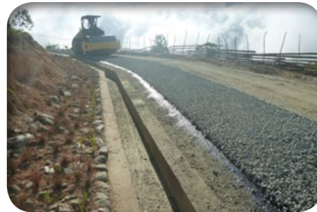
On-going Penetration Macadam work on R4D rehabilitated road Kontinua hala'o hela serbisu Penetrasaun Macadam iha estrada ne'ebé R4D reabilita
