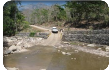
R4D rehabilitated road, Luro-Baricafa (7 km), Lautem District: Example of a level crossing across a wide river and gation protection works Distritu Lautem, R4D reabilita ona estrada Luro-Baricafa (Km 7): Ezemplu nivel paisajen ida korta mota no serbisu proteasaun gabaun
