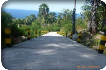
R4D rehabilitated road, Bole-Uatobo (5.2 Km), Baucau District: Concrete pavement on a steep section Distritu Baucau, R4D reabilita ona estrada Bole-Uatobo (Km 5.2): Trotoar ho betuun iha sekaun nai naruk
