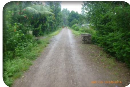
Completed gravel section on R4D rehabilitated road, Bagula-Larisula, Baucau District Kompleta ona seksaun fatuk rahun iha estrada ne'ebé R4D reabilita iha Bagula-Larisula, Distritu Baucau
