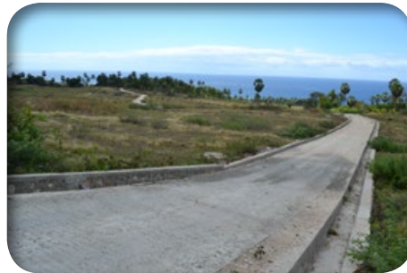
Completed concrete pavement section on the R4D rehabilitated road, Boile-Uatobo, Baucau District Siksaun dalan trotoar ho betaun ne'ebé kompleta ona iha estrada ne'ebé R4D reabilita iha Boile-Uatobo, Distritu Baucau
