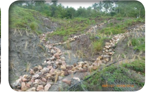
Bio-engineering works, including sub-soil drains, to prevent erosion and landslides Serbisu bio-enjineria, inklui baleta sub solo, hodi prevene erosaun
