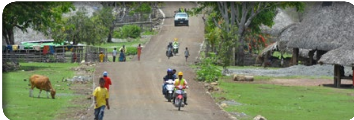
R4D rehabilitated road, Balibo-Cowa (10 Km), Bobonaro District: Another example of concrete pavement on a section with a steep road gradient Distritu Bobonaro, R4D reabilita ona estrada Balibo-Cowa (Km 10): Ezemplu seluk ida husi trotoar betuun iha sekaun ida ho gradienti estrada nai naruk
