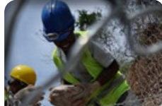
Gloves are also used when labourers are working with stones Uza mos luvas wainhira traballador sira servisu ho fatuk
