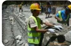
Adequate safety equipment is provided to all labourers according to the specific task they are doing Fornese mos ekipamentu sigur ne'ebé adekuaudu ba traballador hodi tur knaar espesífiku ne'ebé sira hala'o
