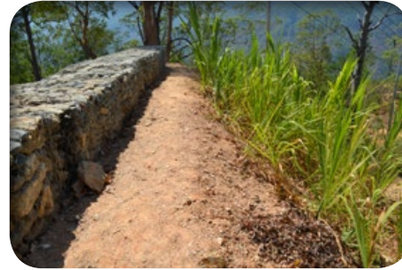
Completed bio-engineering works alongside R4D rehabilitated road Kompleta ona serbisu bio-enjineria iha estrada hirak ne'ebé R4D reabilita ona
