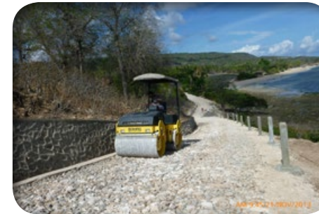
Compaction of Telford base on R4D rehabilitated road, Boile-Uatobo, Baucau District Kompataasaun baze Telford iha estrada ne'ebé R4D reabilita iha Boile-Uatobo, Distritu Baucau
