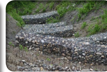
Combination of gabions and bio-engineering to prevent erosion and landslides on steep slopes Kombinasaun gabaun no bio-enjineria hodi prevene erosaun iha rai ho inkilasaun naruk
