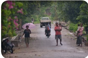
R4D rehabilitated road, Maliana-Sabura (11 km), Bobonaro District: In densely populated areas a proper sealing minimizes dust pollution Distritu Bobonaro, R4D reabilita ona estrada Maliana-Sabura (Km 11): Iha area ne'elebi populasun sira hela barak ku, vedrasun adekuada sei minimiza polusun rai rahun
