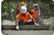
Protective gloves are used for different types of activities, such as working with cement and blumen Luvas protetivo ba tipu atividade oi-oi, hanesan servisu ho simenti no blumen
