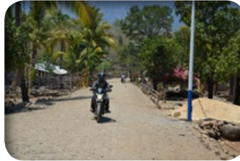
R4D rehabilitated road, Maliana-Sabura (11 km), Bobonaro District: On flat sections often gravel is used Distritu Bobonaro, R4D reabilita ona estrada Maliana-Sabura (Km 11): Iha sekaun kabeer dilaibarak uza dit fatuk rahun
