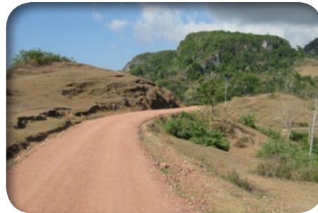
Completed gravel section on R4D maintained road, Caicoli-Liabala, Baucau District Kompleta ona seksaun ho fatuk rahun iha estrada ne'ebé R4D halo manutensaun iha Caicoli-Liabala, Distritu Baucau
