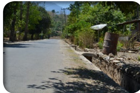
Completed Penetration Macadam section on R4D rehabilitated road, Maliana-Saburai, Bobonaro District Kompleta ona seksaun Penetrasaun Macadam iha estrada ne'ebé R4D reabilita iha Maliana-Saburai, Distritu Bobonaro
