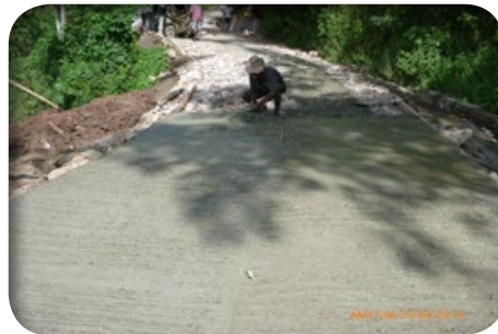
On-going concrete pavement work on R4D rehabilitated road Sei kontinua hala'o hela estrada trotoar ho betaun iha estrada R4D nian
