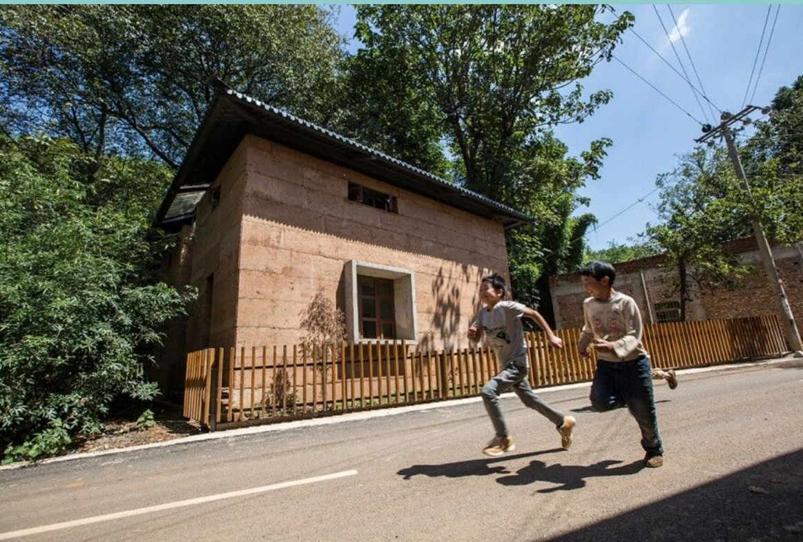
Rammed-earth-earthquake-resistant house - China
