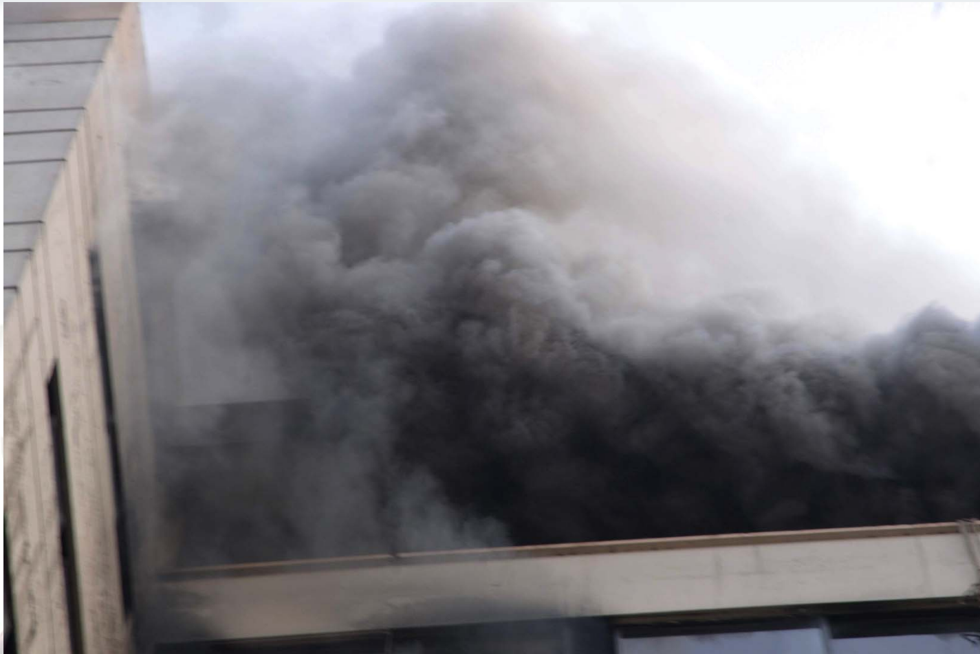
Fire Hazard (Smoke )
