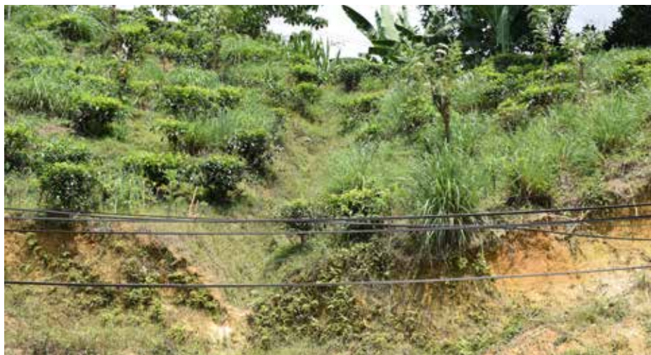
Figure 3.10: Lack of proper drainage systems observed in tea lands (Source: EFL)
