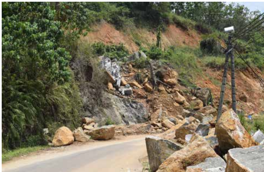
Figure 3.1: Ongoing landslide alongside Ratnapura-Wewalwatta road (Source: EFL)
