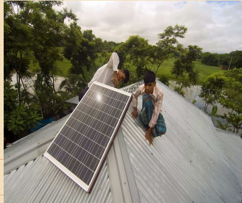
Solar Installation in a rural house
