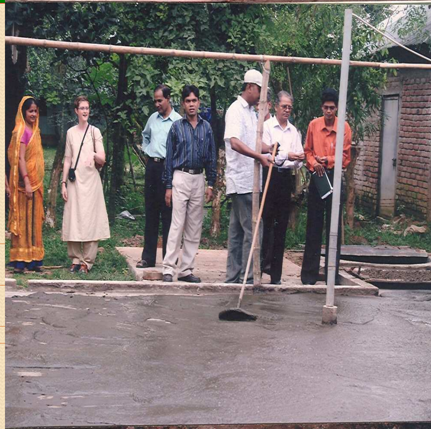
Slurry Processing at a biogas plant
