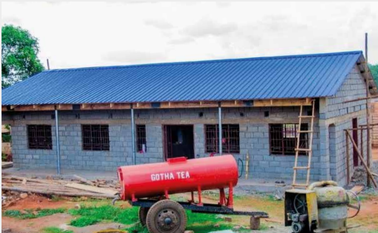
A victim support unit under construction, supported by a tea estate at Thyolo Police Station in Thyolo District.
