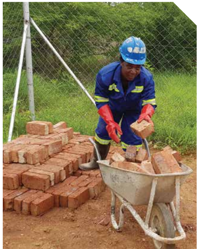
Beneficiary of YWEP engaged in the construction of the Tomato Paste Factory
