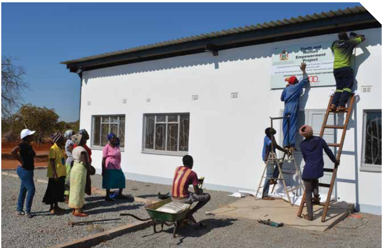
Rovhona Raita Horticulture Cooperative members supervising the mounting of the project signage on the front wall of the Mopane Worms Processing Factory in Beitbridge
