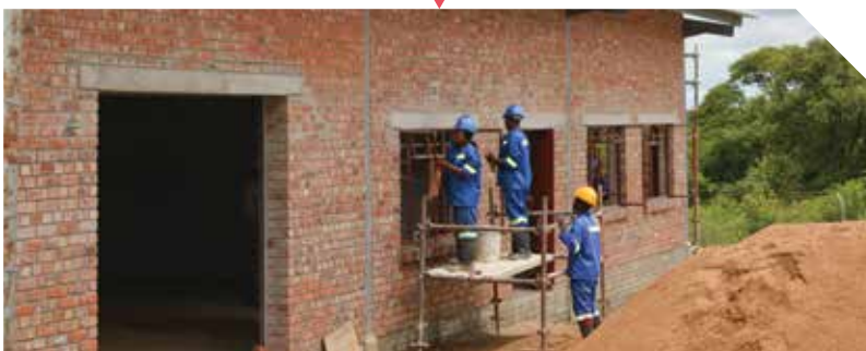
Tomato Paste Processing Factory under construction
