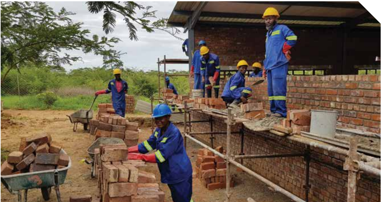
Beneficiaries of YWEP engaged in the construction of the Tomato Paste Factory
