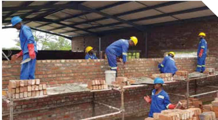
Construction of the Tomato Paste Processing Factory by Youth in Mutoko
