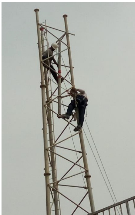
► Figure 4-3. Actual Snapshot of rooftop site buildup operations
