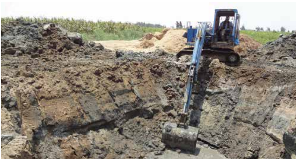
Dredger carries out excavation work at the site of the Biogas digester unit.
