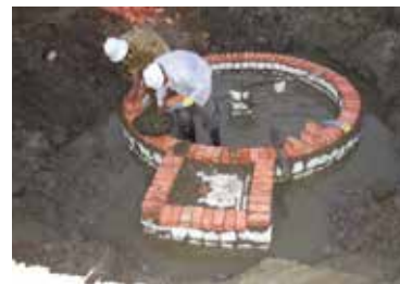
Subsurface work at the site of the Biogas digester unit.
