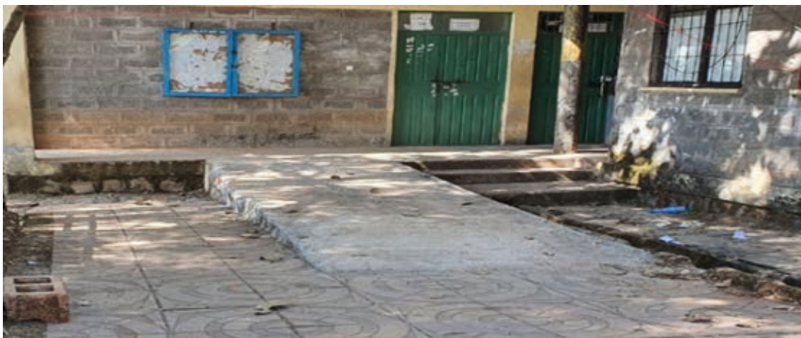
Figure 27: A classroom improved to make it accessible for physically challenged persons
