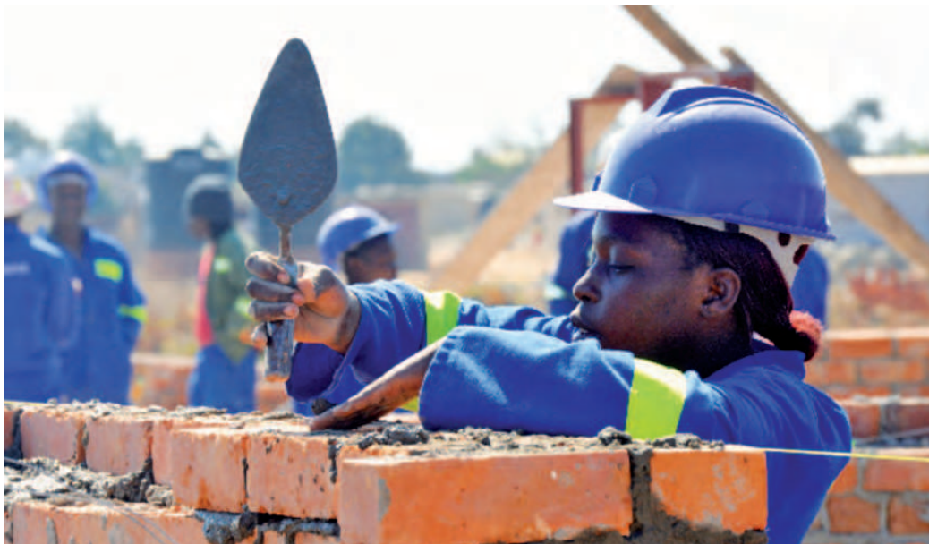
On-the-job training in brick-laying
