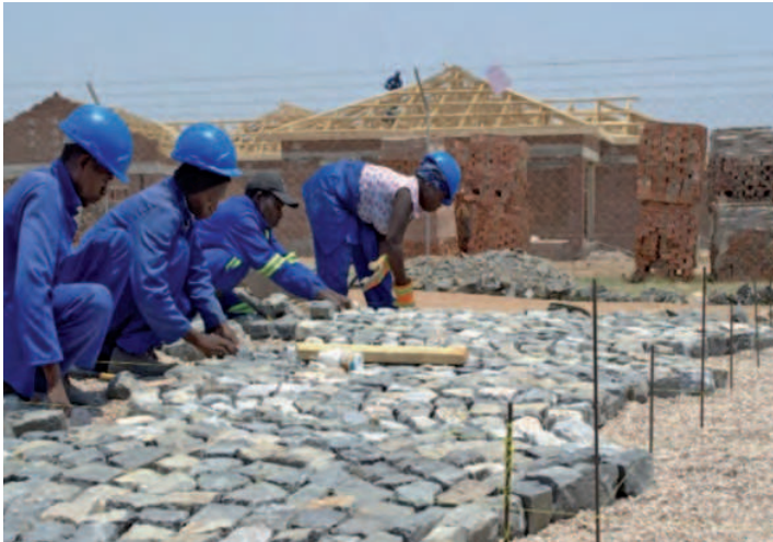
On-the-job training in cobble stone paving
