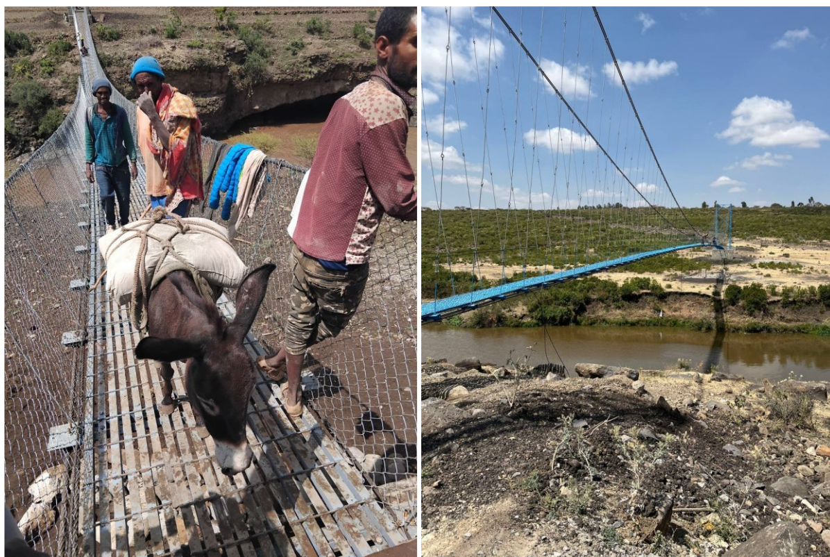
► Figure 24. Suspended Bridge over Tekeze river (left) & Suspension bridge over Akaki river (right)
