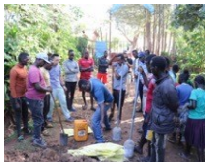
► Figure 8. Repair work in cooperation with residents.
