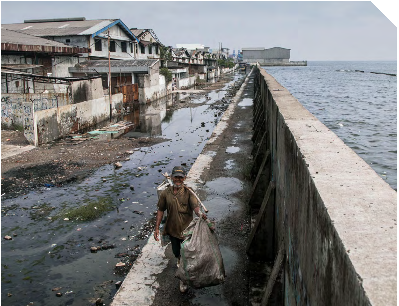
Behind the wall, a man walking on top of a giant sea wall protecting Jakarta, Indonesia, 2021. ©Climate Visuals Countdown/Irene Barlian
