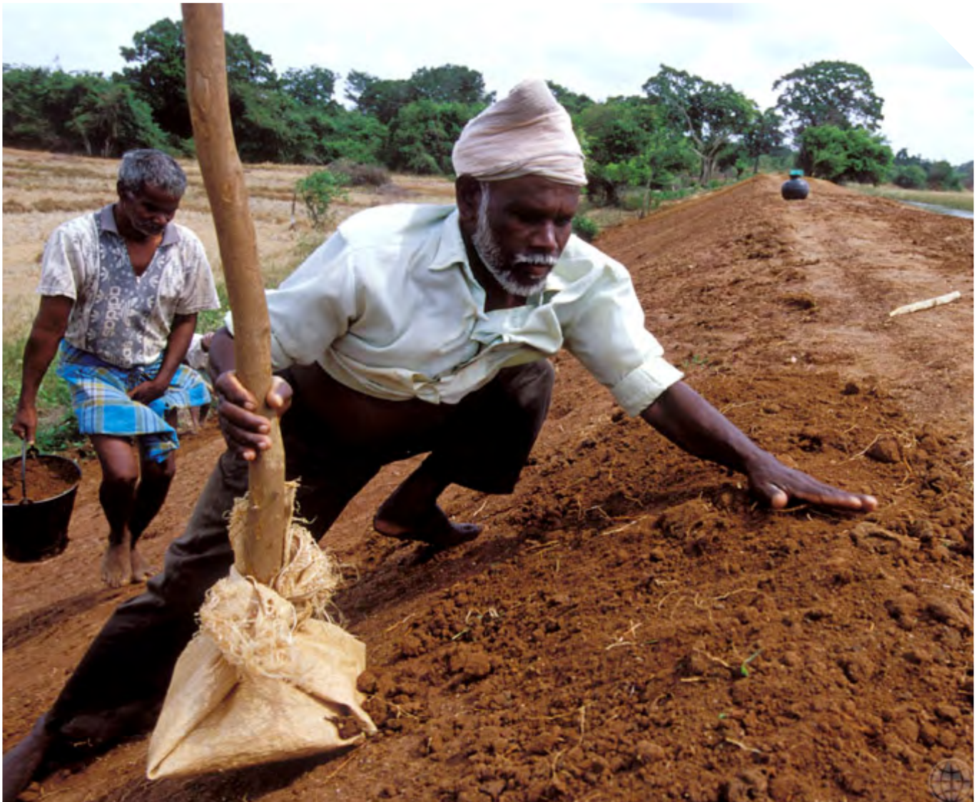
Flood protection. Two men work on repairing and refilling breached sections of embankments, Sri Lanka, 2007. ©World Bank/D. Sansoni
