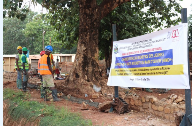
Training demonstration site for labour-intensive infrastructure works under the EIIP project. Central African Republic, 06/2019 © ILO
