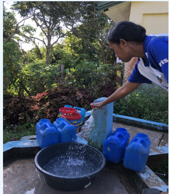
Water supply facility constructed under the ILO-Japan Water Project in BARMM, Philippines, 2023. @ Arvy Origenes/ILO
