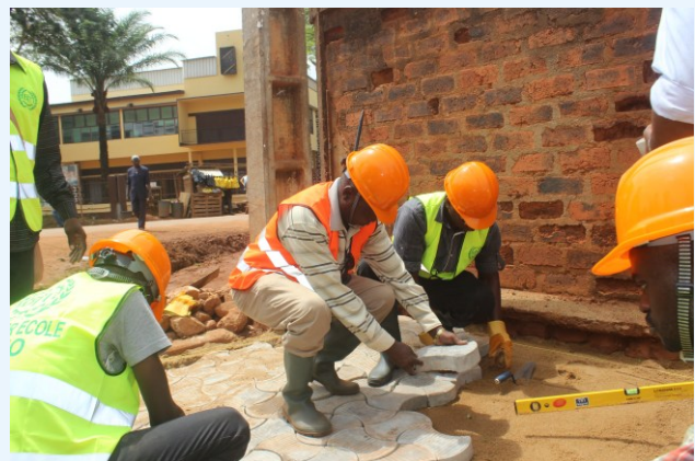
On-the-job training in paving block installation under the EIIP project. Central African Republic. © ILO
