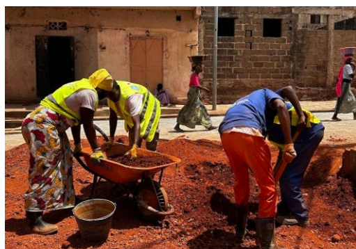
Workers carrying out urban road improvement works using STEIN in Bamako, Mali, EIIP Project, March 2026. © ILO
