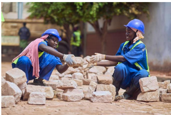
Women carrying out road works, ZNRY, Bamako, Mali, EIIP Project, March 2026. © ILO
