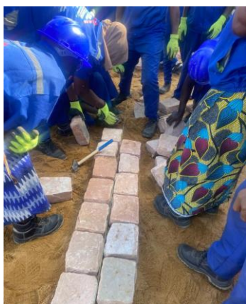
Practical training as part of the chantier école, CFP Sénou, Bamako, Mali, EIIP Project, December 2025. © ILO
