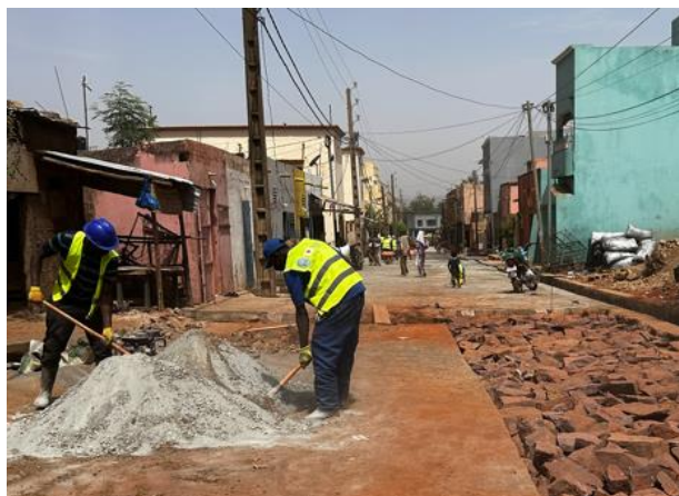
Road improvement works, ZNRY, Bamako, Mali, EIIP Project, March 2026. © ILO
